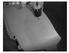
**STEP 7:** Use the remaining mounting holes as a drill guide.
