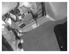
**STEP 10:** Using a 1/2" drill bit, drill a hole through the metal floor in the location of the impression in the wax square.
